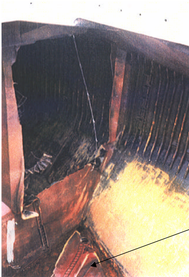
Photograph 1 Collapsed and detached transverse bulkhead
