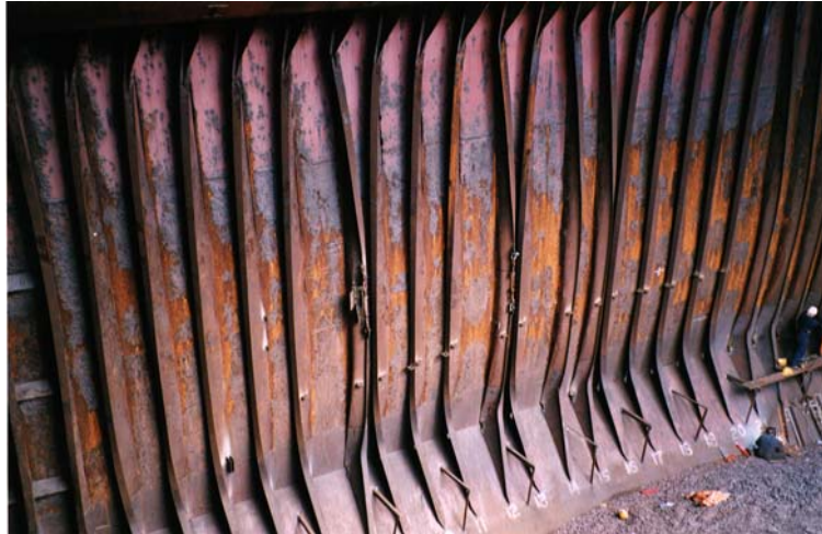
Photograph 1 Collapsed side shell frames (See Example 4)
