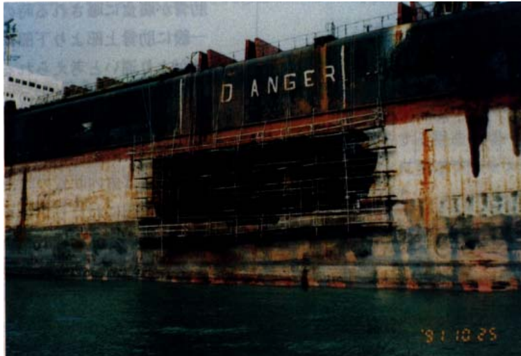
Photograph 2 Missing side shell structure (See Examples 4 and 5)
